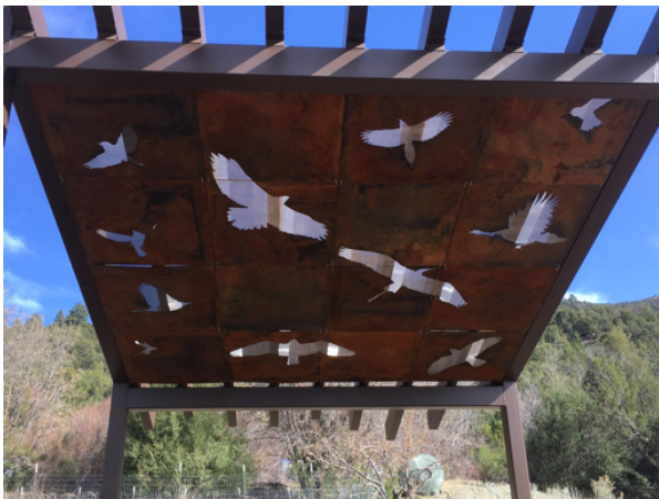
The solar shade at Randall Davey Audubon Center, funded by a donation from Tom and Carlyn Jervis. Birders can find respite from the sun beneath, while photovoltaic panels on the top generate electricity for the center's David J. Henderson Pavilion.
