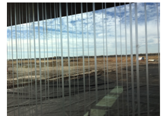
Etched lines on bird-friendly glass
