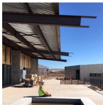
A view from outside the almost-finished center
